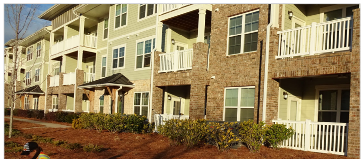
A multistory residential receptor with outdoor use areas (porches and balconies) in the PSA.
